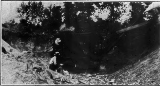
Steam Shovel Stripping Loam from The Surface
